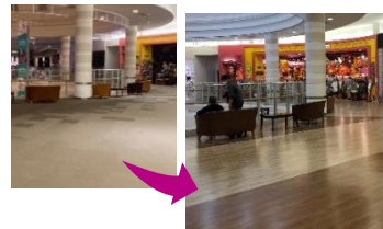
Floor replacement work
