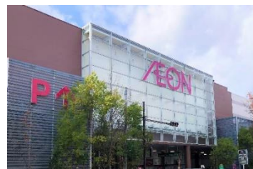
Exterior wall painting
