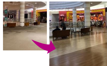
Floor replacement work
