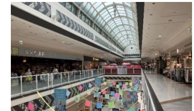
Refurbishment of ceiling top lights
